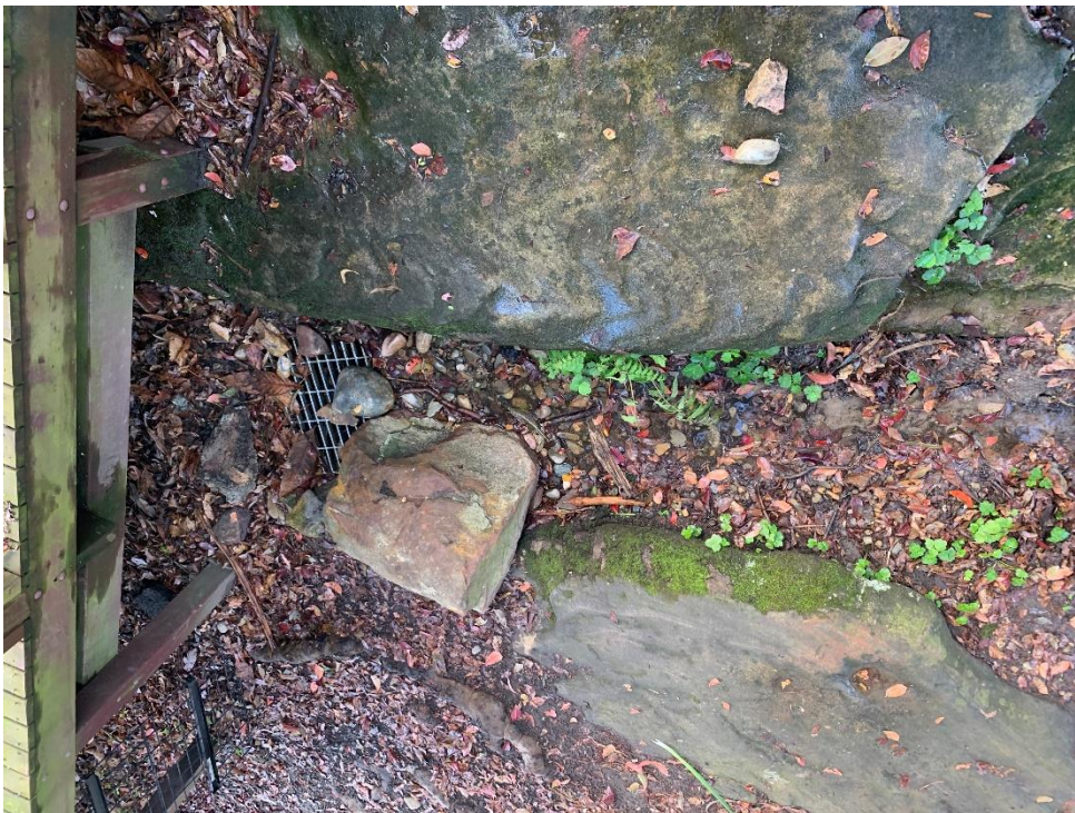
Figure 4.26 Water source diverted to stormwater drain. Located on the lower slope. AMAC Group, IMG 5903 (18/08/2023).
